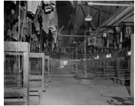
View showing miners' clothes suspended by pulleys, also wash basins and ventilation system, Kirkland Lake, Ontario, 1936.
