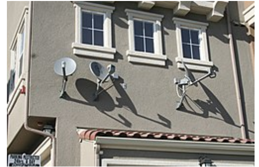
DBS satellite dishes installed on an apartment complex.
