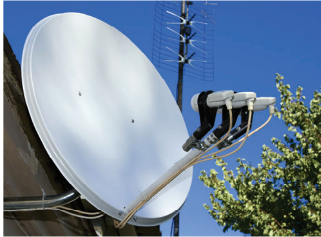
Figure 75. Dish antenna with multiple LNBs.
