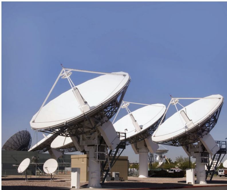
Figure 63. Cassegrain uplink antennas for television broadcasting.
