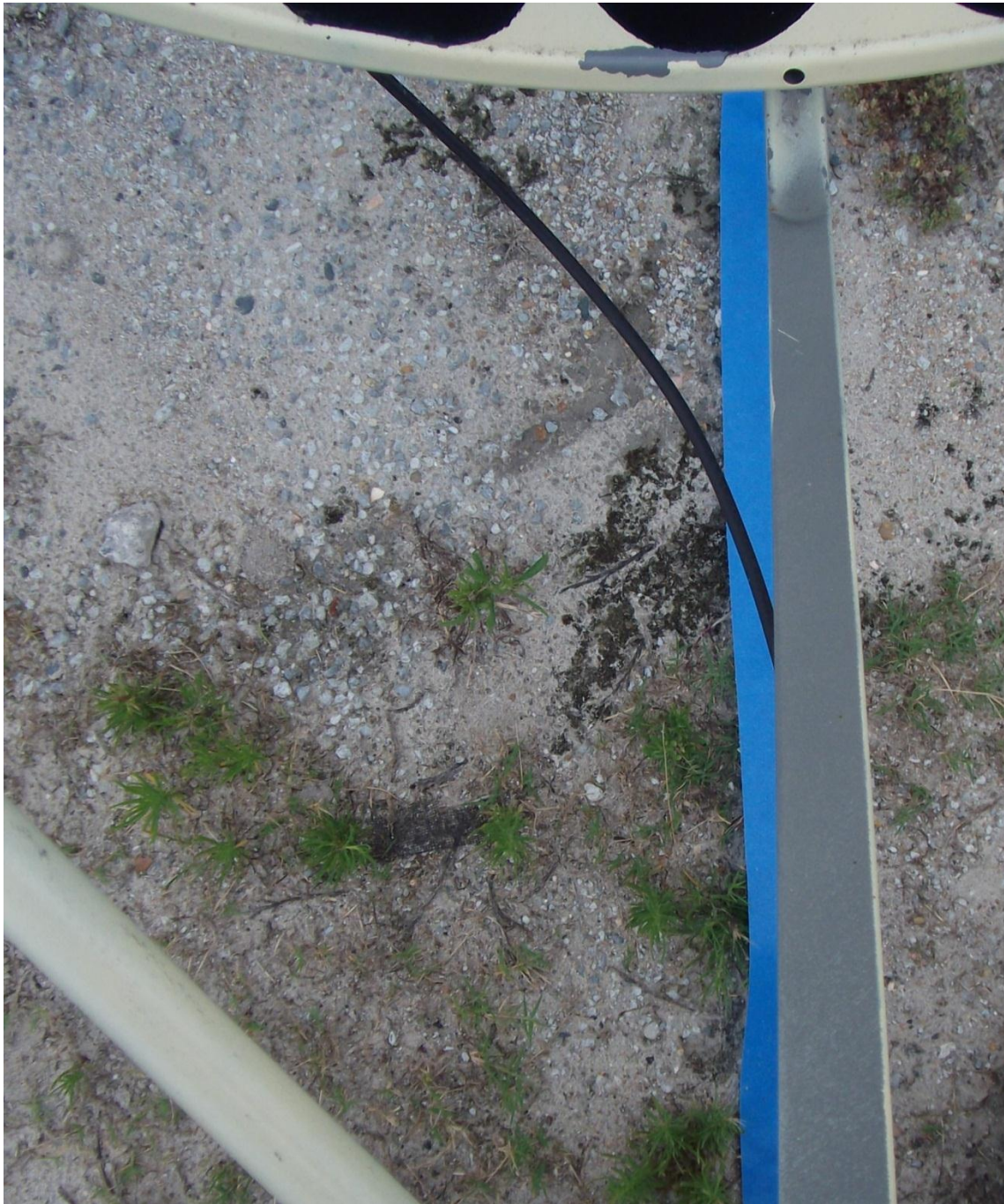
Figure 9: Align LNB mounting arm to north-south line.
