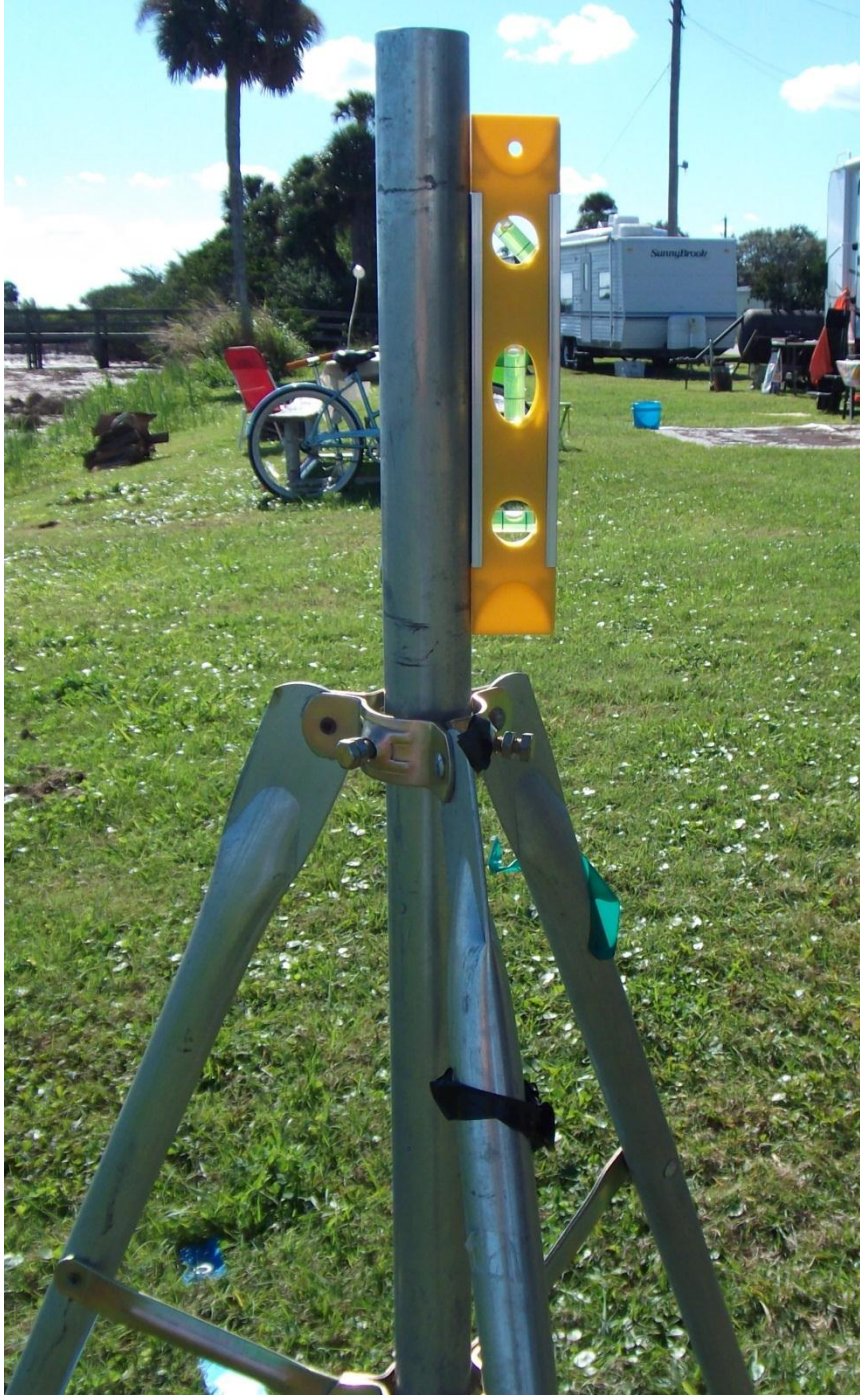
Figure 7: Checking for vertical alignment with a level
