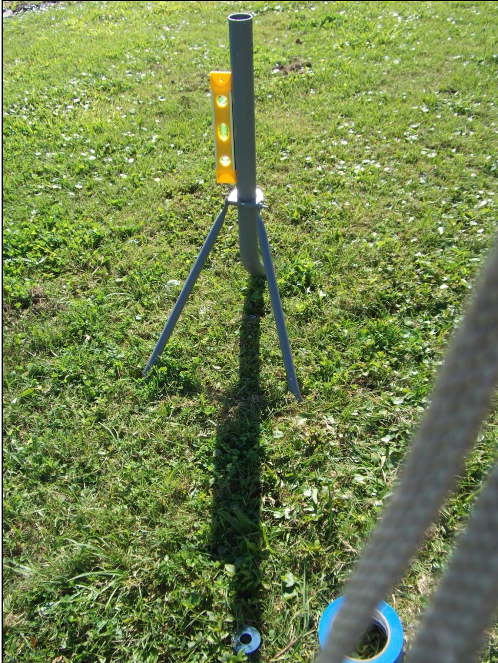
Figure 3 Location for center of dish motor mounting mast is marked by fender washer.
