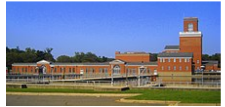
Dalecarlia Water Treatment Plant, Washington, D.C.
