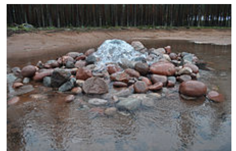
At Turun Seudun Vesi Oy's artificial groundwater plant , the pretreated raw water from the Kokemäki River is absorbed through the basins into the Virttaankangas ridge formation.
